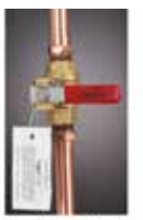
Water Shut off valve
